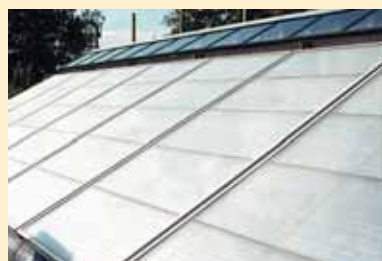
With PVT, solar energy is converted to heat and power simultaneously in one device. (Photographs: ECN, Vattenfall, ECN)
